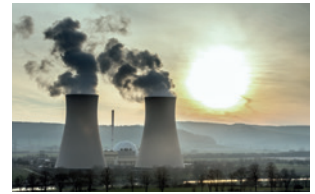
Power station cooling towers
