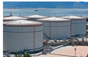
Tanks and containers
