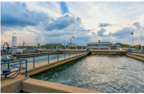
Collecting and retaining basins
