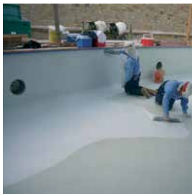
Trowel application under tiles
